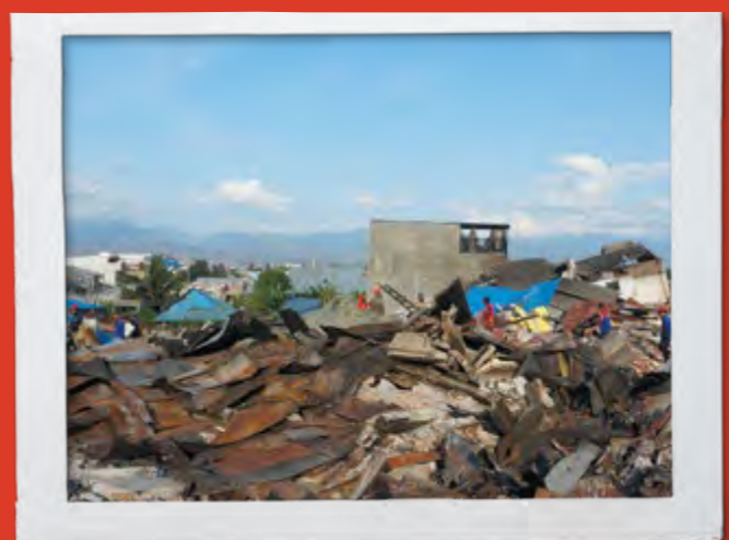
In the Palu neighborhood of the Indonesian island of Sulawesi, about 1700 houses were swallowed up when the earthquake caused soil to liquefy. Photo: Ade Nuriadin, Catholic Relief Services, (CRS)
